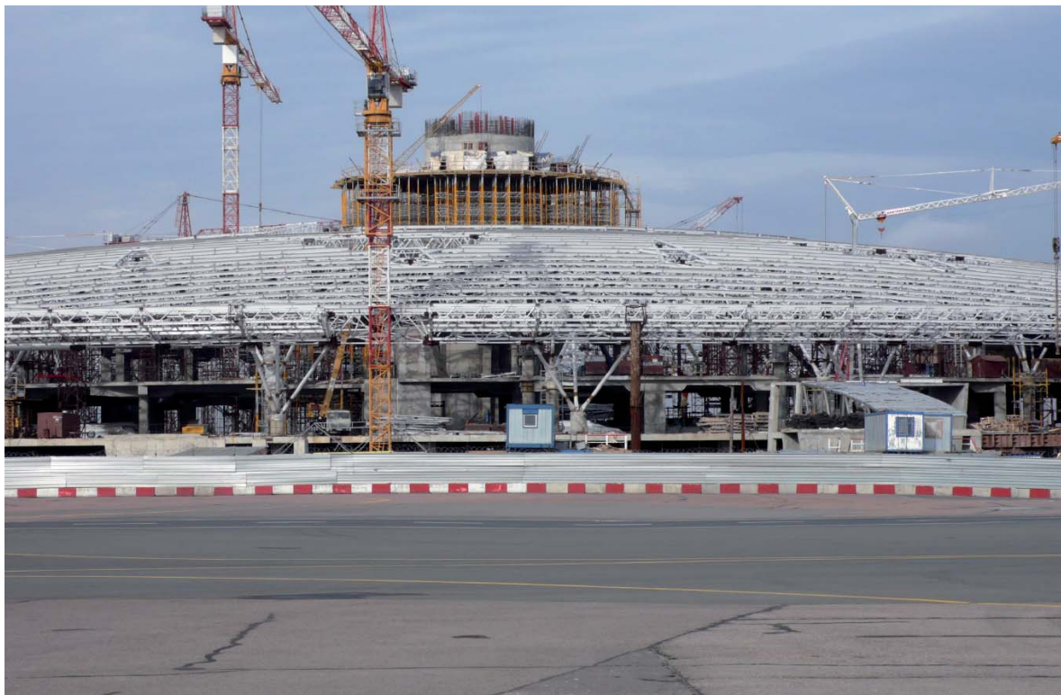
Building site of airport Moscow Vnukovo
